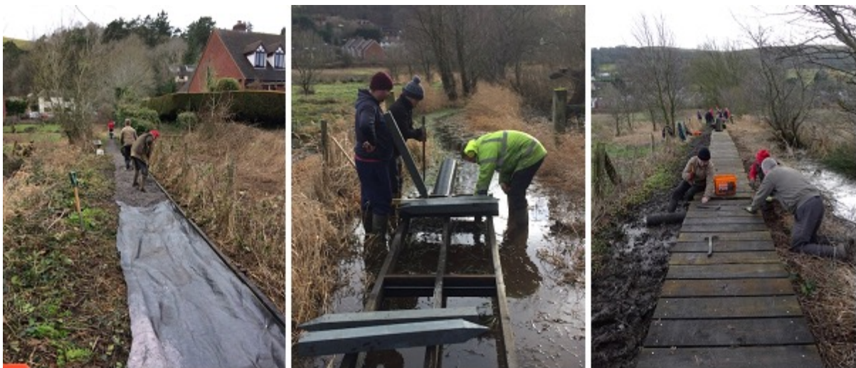
Figure 10: Installation of the boardwalk
